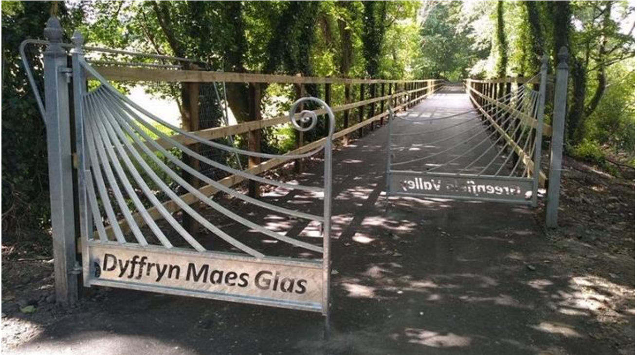
Figure 4-4: Staggered Gates Example 1 - Holywell, Flintshire
